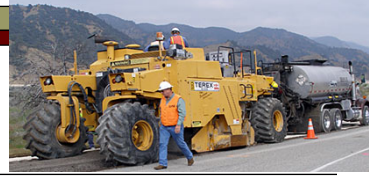
Full Depth Reclamation
