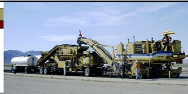
Cold In-place Recycling
